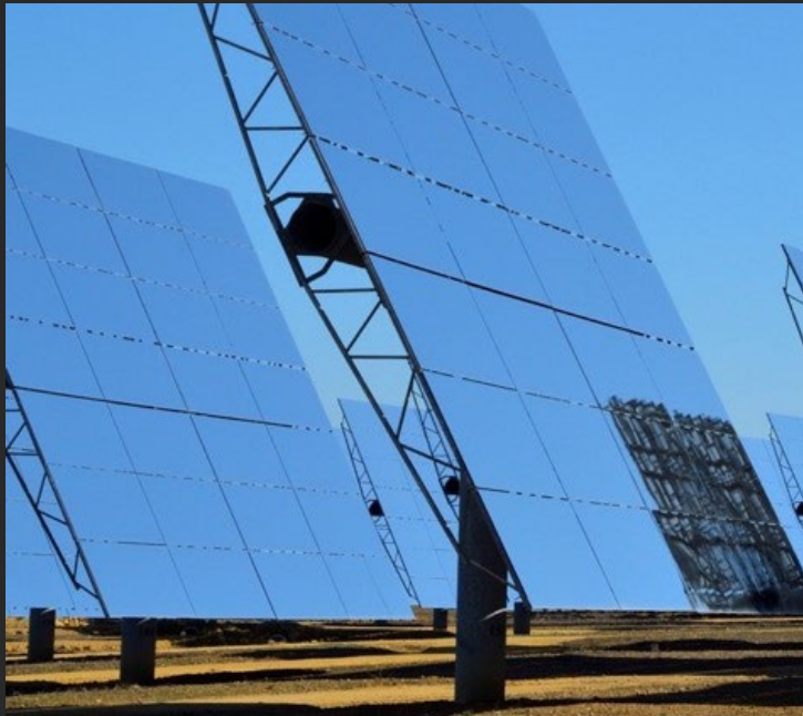
MI Energy Solutions Solar Panel Repurpose & Recycling
