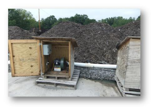
• Air is injected into the piles via the piping network, accelerating the decomposition process and eliminating the need to routinely turn the pile.
